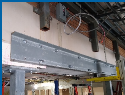
Begin Install of Support Steel in Cafeteria
